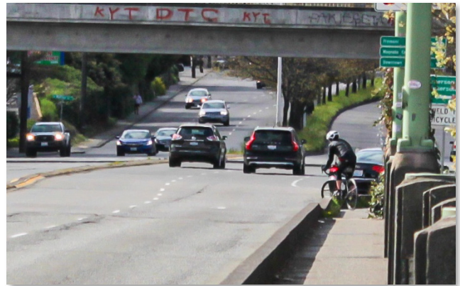
Challenging merge for southbound bicyclists at 15 th Avenue W & W Emerson Street
