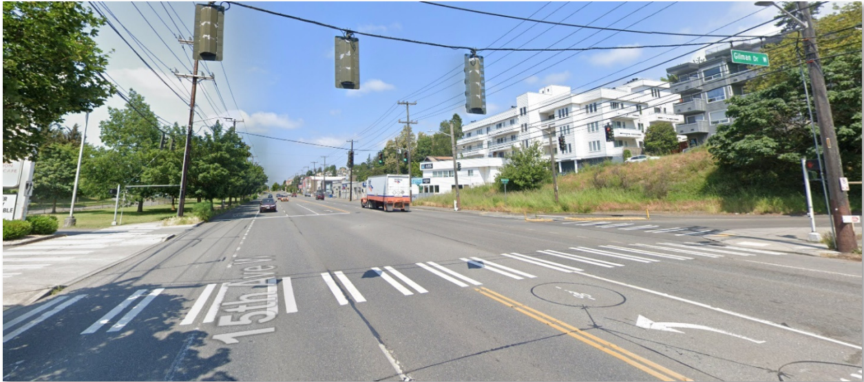
Figure 23: 15 th Avenue W at Gilman Drive W, looking north
